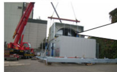
In 2007, we delivered the world's biggest desiccant dehumidifier rotor* with 4500mm in diameter and 400mm in depth (*as of October 2008)
